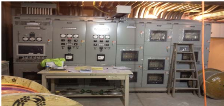
PARALLELING SWITCHGEAR
